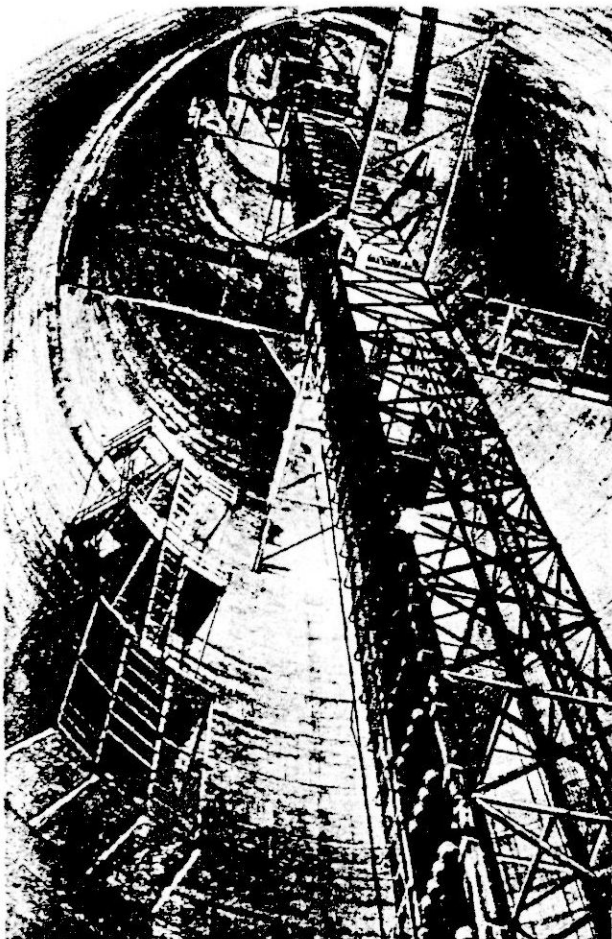
Fig 6. Lift cage and internal platforms
